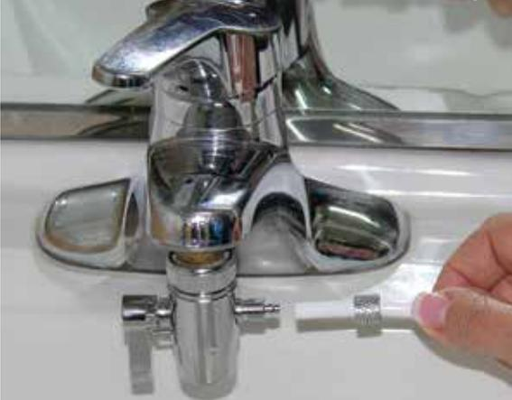
**1. ATTACH DIVERTER TO YOUR TAP** - Remove the aerator from tap (pliers may be required) and attach diverter valve in its place. There are adapters supplied in case the diverter does not fit your tap. If you have leaks at the diverter, use plumber's Teflon tape (included).
